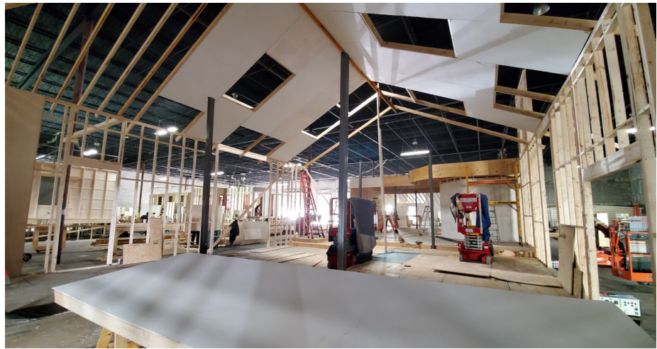
Construction build in progress.
